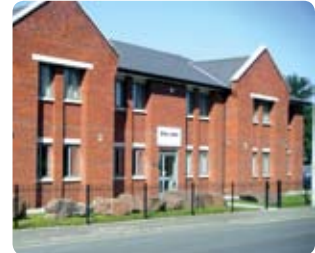
SitexOrbis Alarm Receiving Centre, Wirrel, UK. BS5979 Cat II and BS8484 accredited centre.
